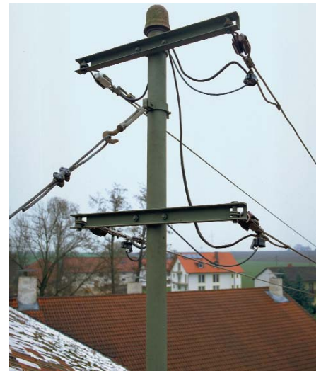
Service entry through overhead system
