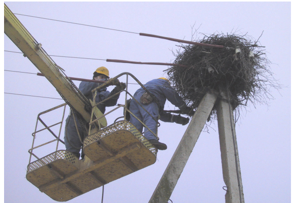
Pilt 2. MVLC paigaldamine
