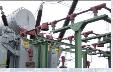
Substation equipment is vulnerable to flashovers caused by accidental bridging of phases, or phase to earth. Usually made by birds, animals, vegetation or airborne debris, flashovers can be very expensive in terms of damage to equipment, reduced reliability and in some cases even electrocution of protected species.
